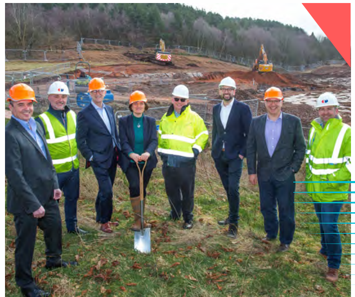
Groundbreaking ceremony to celebrate construction of the new Supercomputing Centre at Daresbury Laboratory, February 2023
